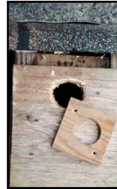
Repairing the hole size
