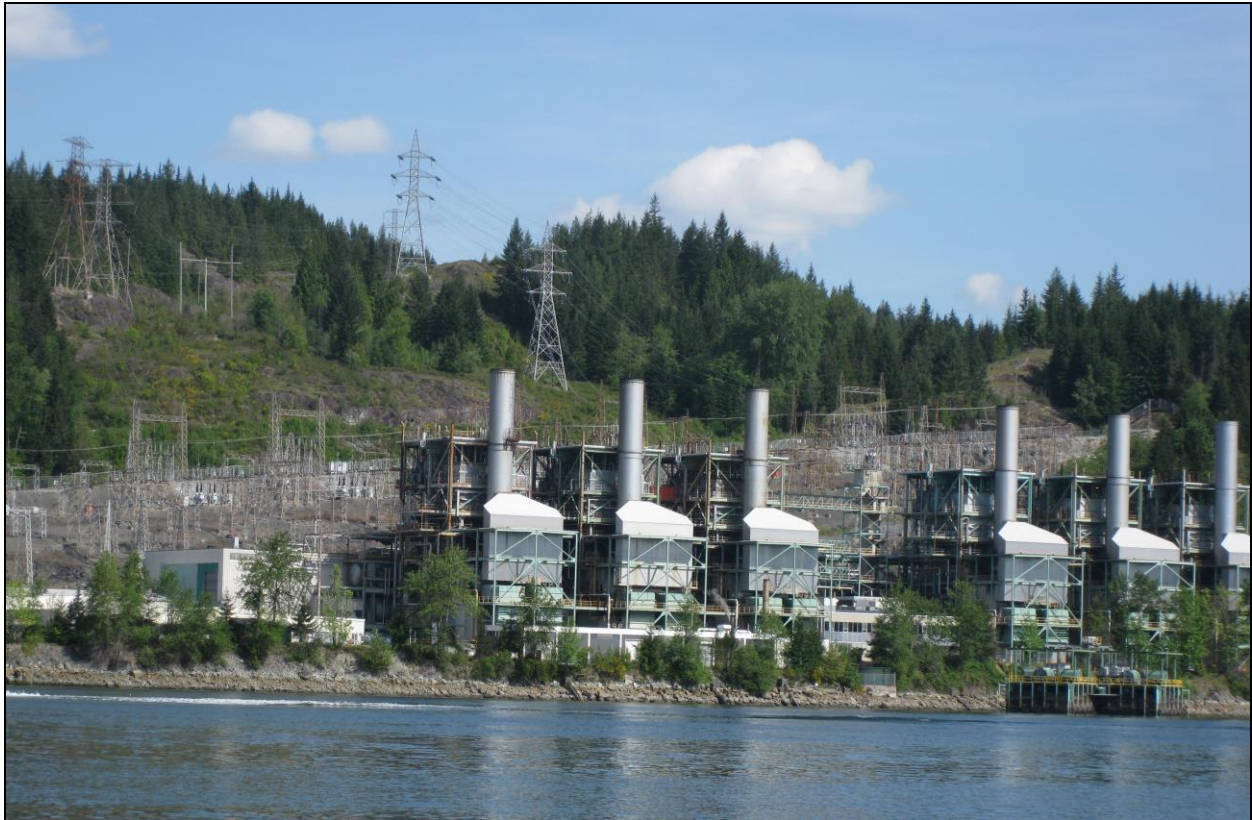
The Burrard Thermal plant on the north shore of Moody Arm. V. Otton photo.
