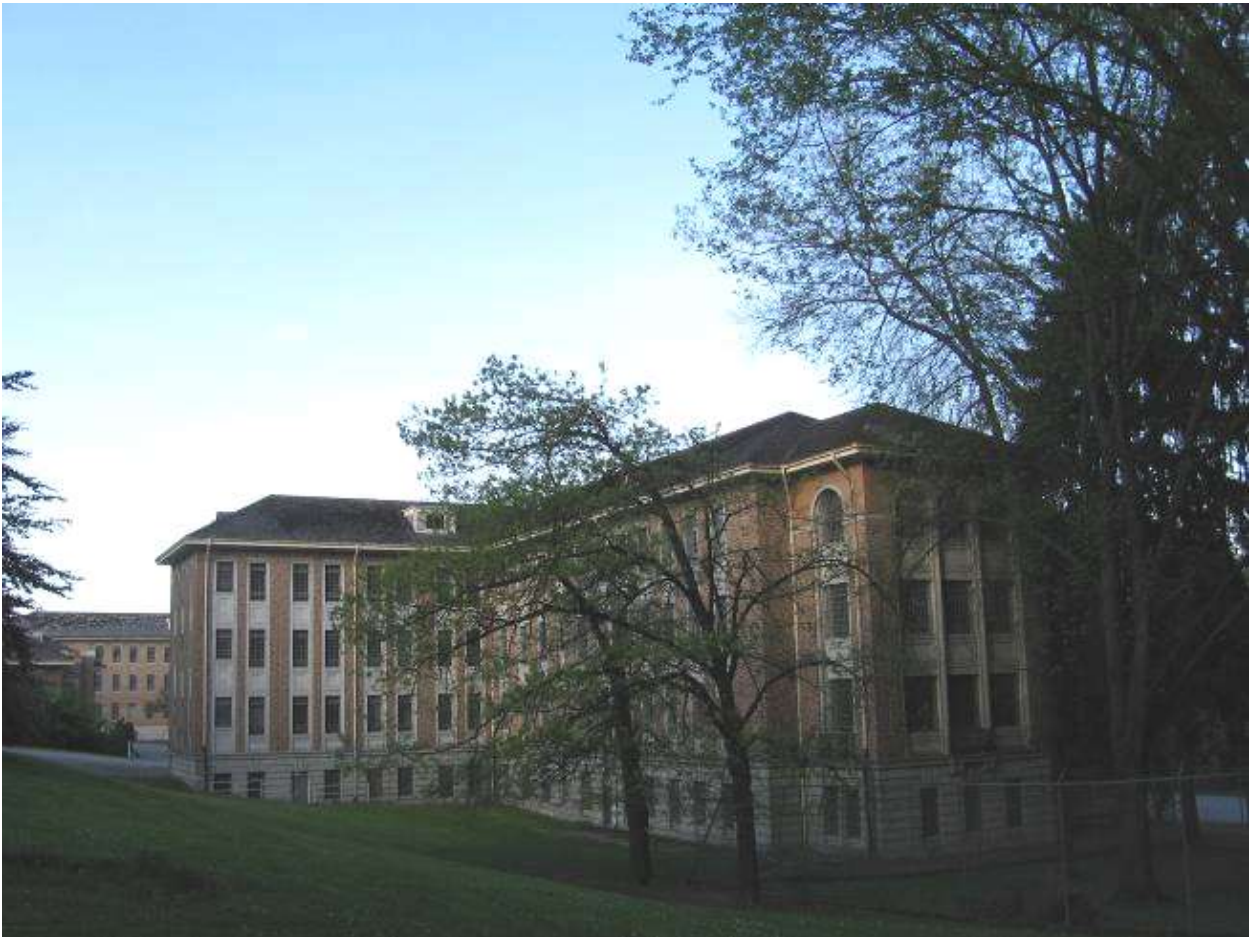
The Crease Clinic, an excellent example of the Art Deco period, now has a new roof and has been used by the film industry for many years. Despite this, its condition is assessed as "critical". Photo Credit: Niall Williams.
